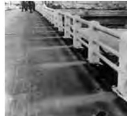
Shadow of railings on the bridge floor of the Yorozyu Bridge. It remained white where the rays were blocked by the railings. (from US Forces B-105)
