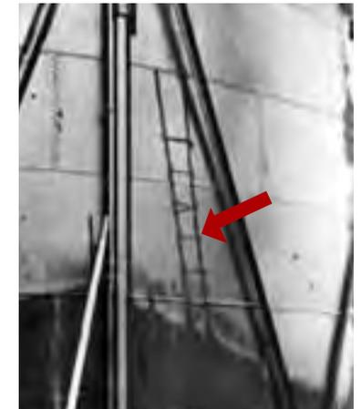
A roof and ladder etched on a gas tank where they were in shadow retained their original black color. (from US Forces B-127)
